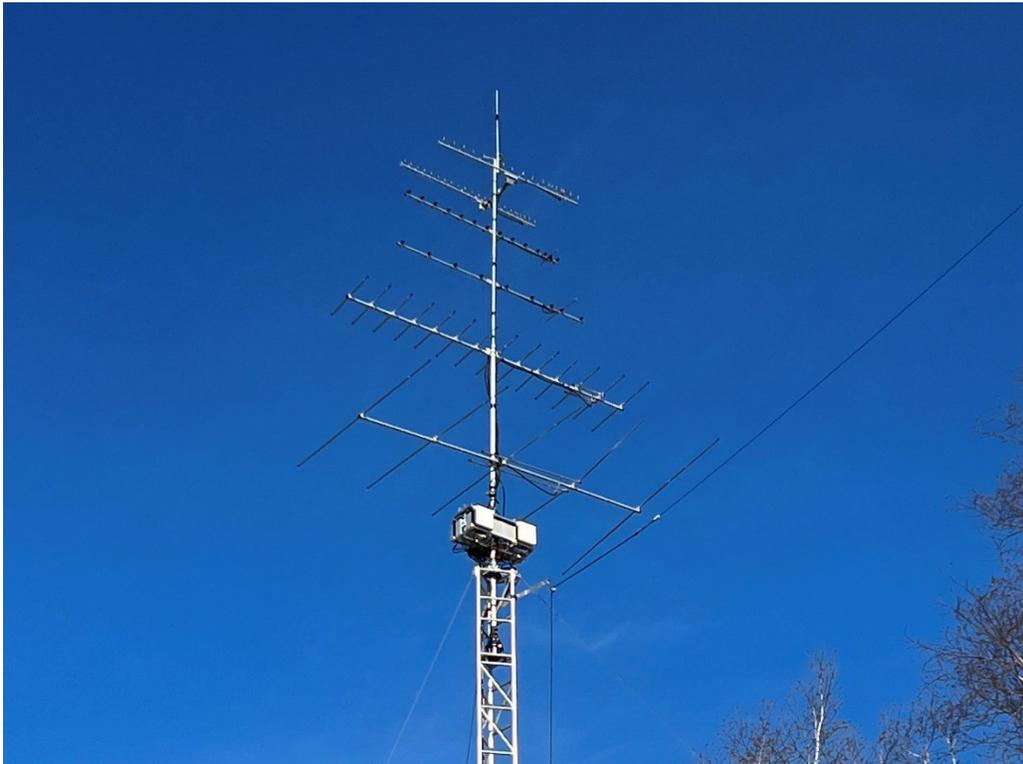
Antennas, amplifiers and LNAs for 50MHz thru 1296MHz at K1UU
